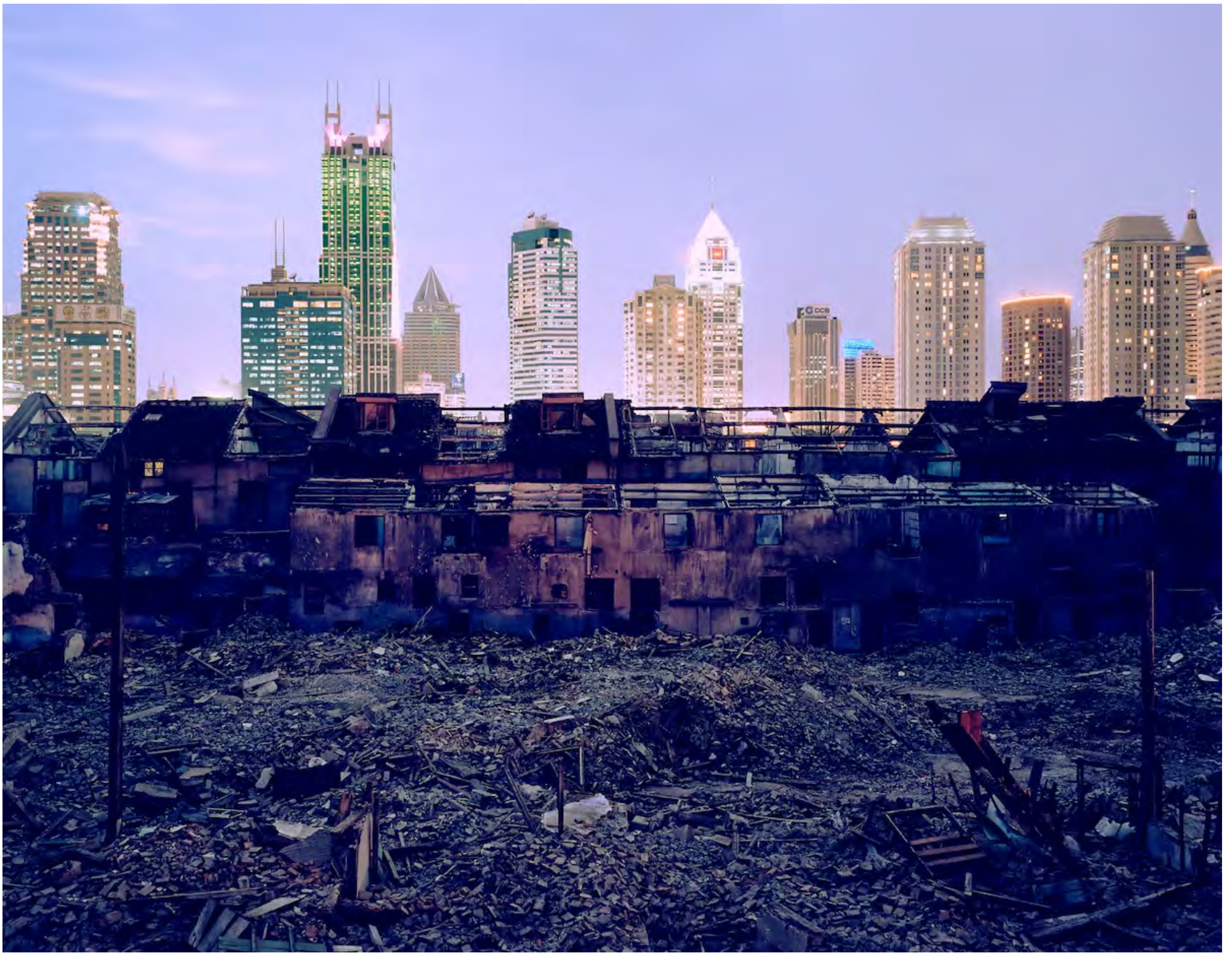
Shanghai Falling (Fuxing Lu Neighborhood Demolition), 2002.
